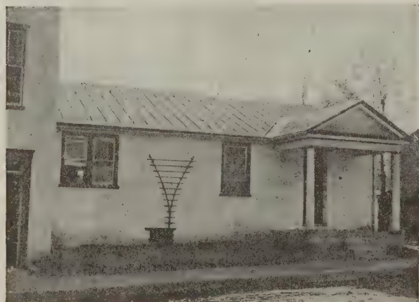
Old school house converted into a bungalow. The original building had walls of whitewashed stone. Opening to the left was originally a single window, which has been enlarged. The porch is new. Roof is of tin laid with standing seam
